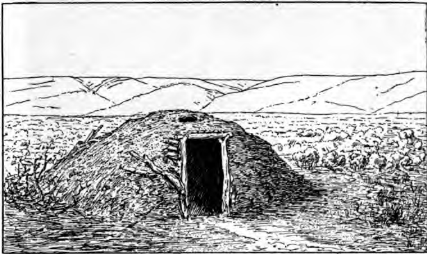
FIG. 240—Low earth-covered shelter
